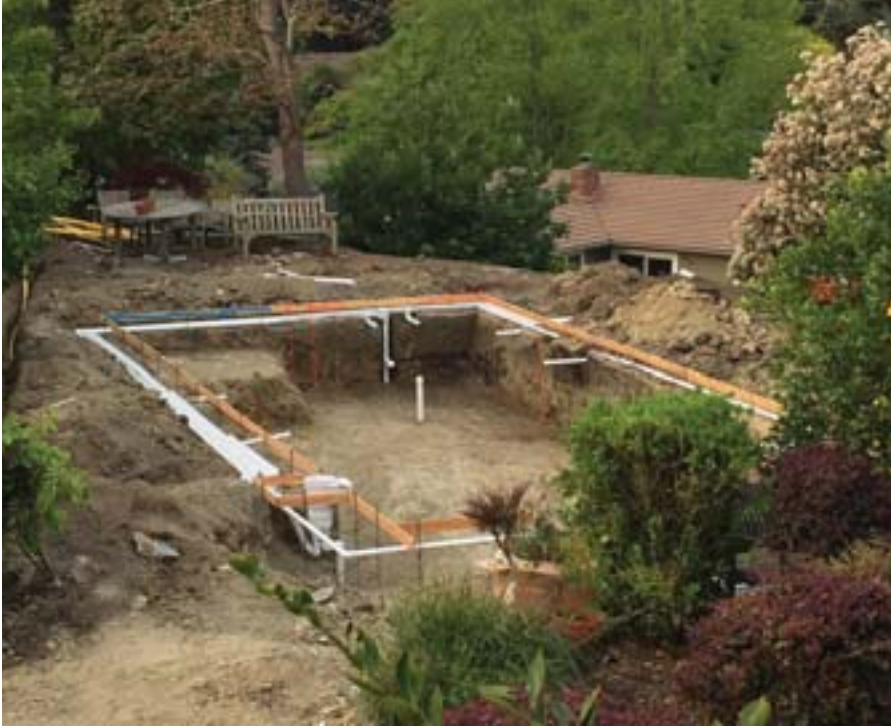
Pool dug to 6.5-foot depth; circulation pipes installed.
